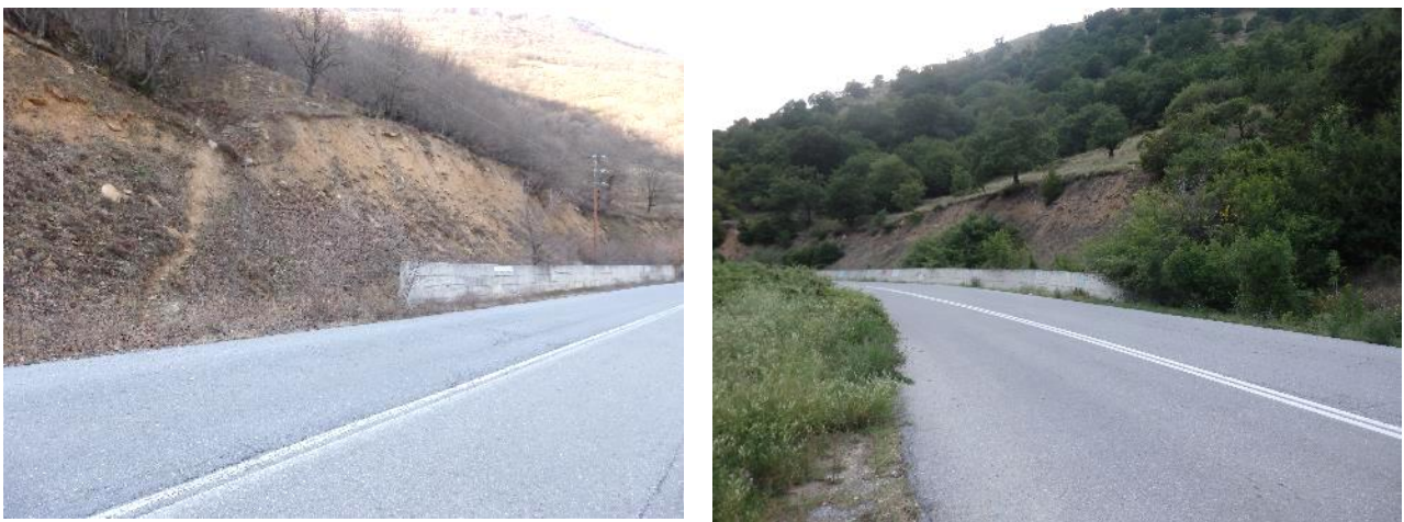
Figures 37 Supporting road walls act as barriers to wildlife movements but when combined with good crossing habitat funnel animals at their edges to create hot spot crossing points (Aetos-Sklethro road segment). Note the bear /wildlife path at the left picture.
