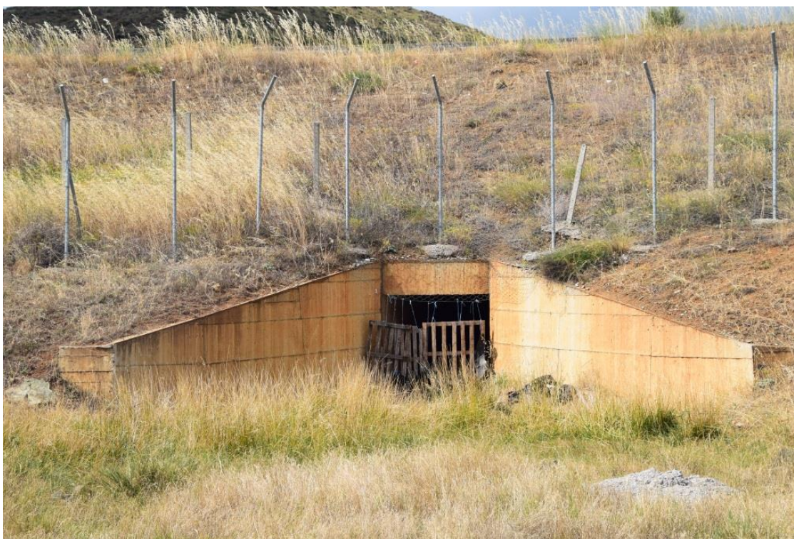
Photo 8. K114 SW entrance. Main intervention: Plantings and removing the obstacles and the debris.
