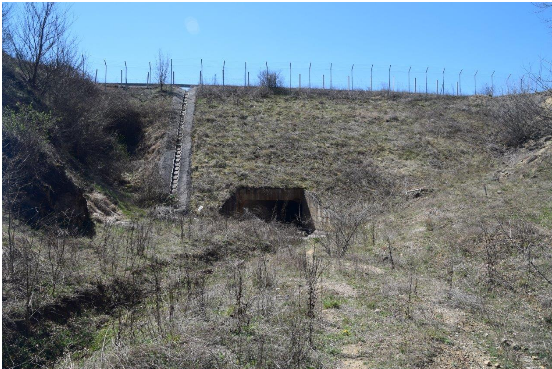
Photo 3. K32, NE entrance. Main intervention: Debris removal and plantings.
