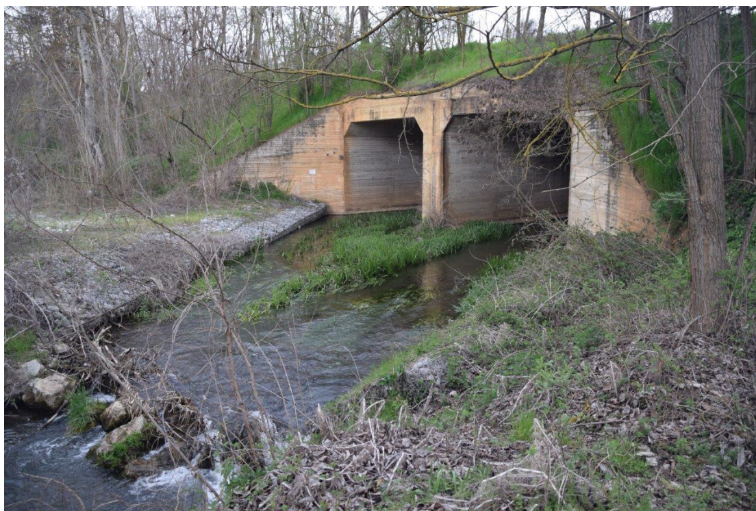
Photo 5a. K74 SW entrance. Main intervention: Creation of dry ledges
