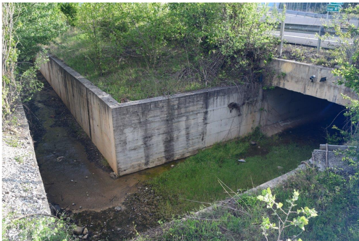
Photo 10. K138 NE entrance. Main intervention: Creating a ramp and install a light/noise screen.
