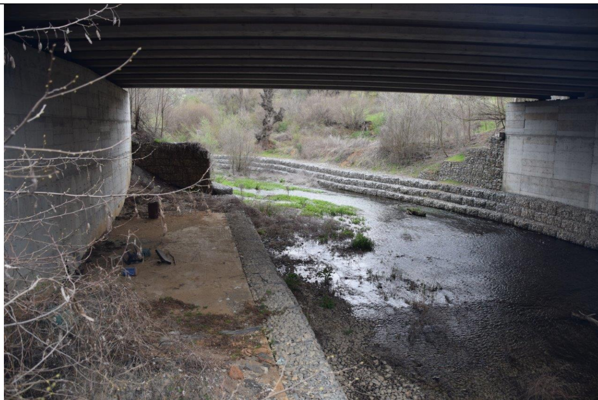
Photo 5b. K74 NE entrance. Main intervention: Continue dry ledges to the SW entrance (ph.5a).
