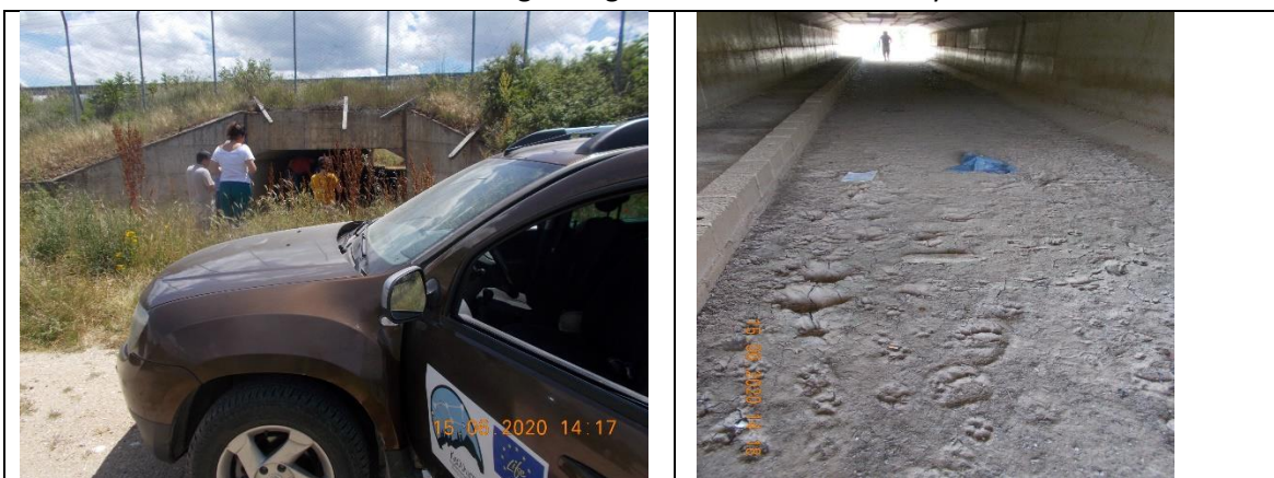
Fotos 3.3.3/2-3: collective field visit of underpasses in June 2020 by all involved project partners
