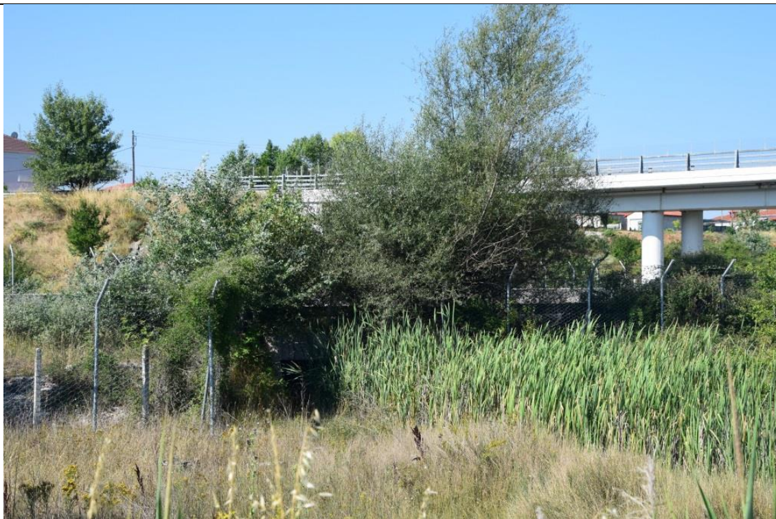
Photo 9. K128b NE entrance. Main intervention: Removing the debris and the vegetation.
