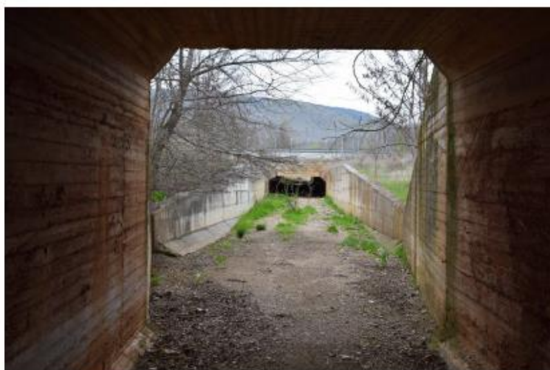
Photo Entrance 1:SW
