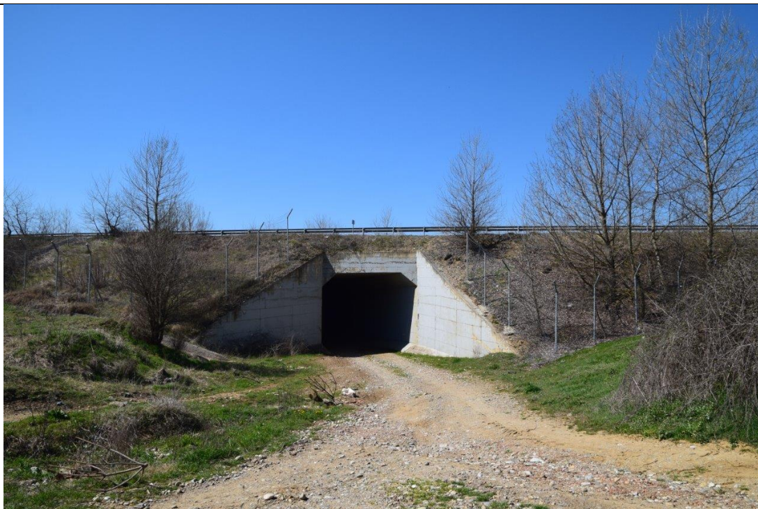
Photo 4. K46 NE entrance. Main intervention: Correction of the fence ending on the sides and plantings.
