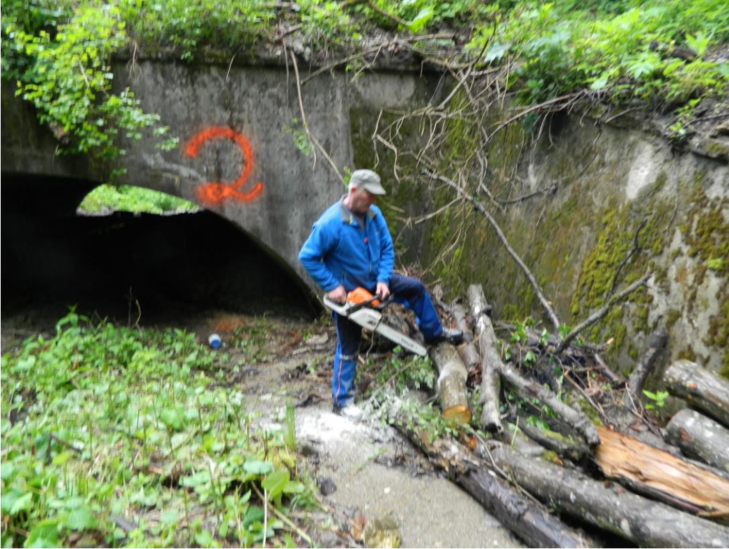
Figure 5. Intervention carried out at the selected crossing structures.
