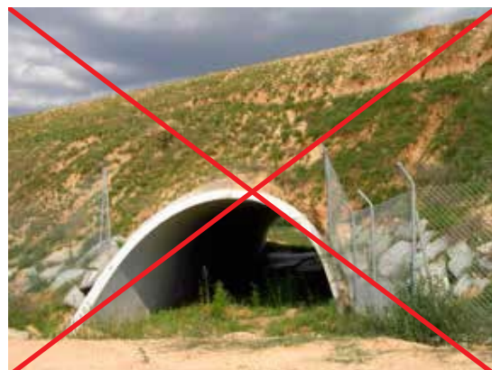
Figure 6.10. Incorrect fencing of the underpass walls permits animal access to the embankment. Photo: C. Rosell.
