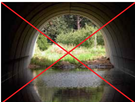
Figure 6.9. Flooded underpass base hinders its use by wildlife. Photo: C. Rosell.
