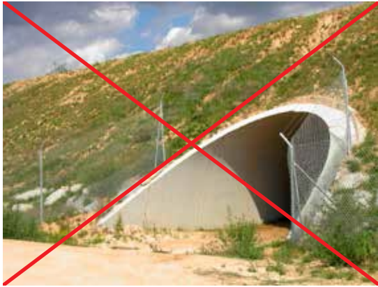
Figure 13.10. The fence should lead to the crossing, leaving no gaps that permit entrance to the embankment. Photo: C. Rosell.
