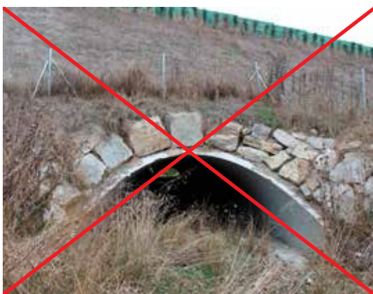
Figure 12.7. Incorrect installation of a perimeter fence, which does not guide animals towards the crossing entrance. Photo: M. Fernández-Bou.
