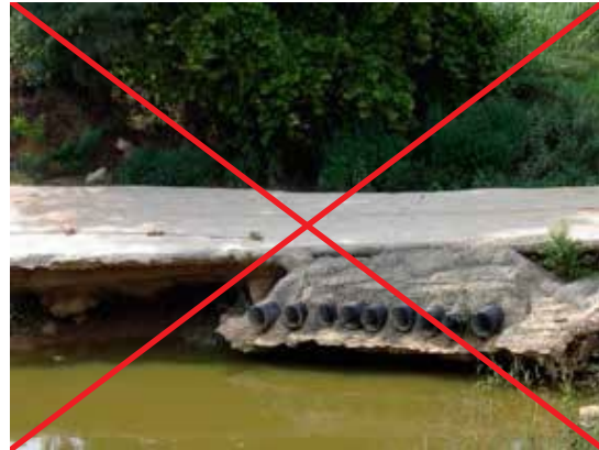
Figure 5.6. Works track that has interrupted the continuity of the watercourse. Photo: R. Campeny.
