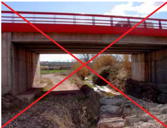
Figure 7.7. Riprap hinders the passage of wildlife. Photo: F. Navàs.
