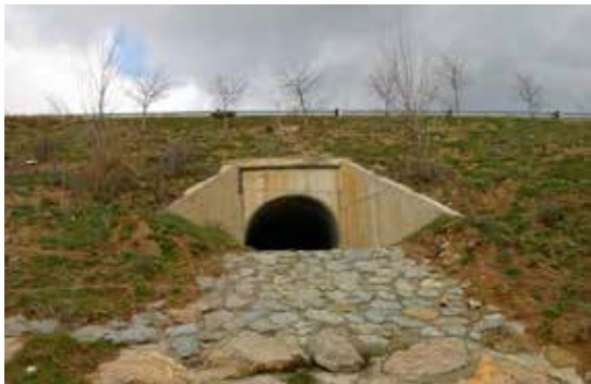
Figure 9.7. Stone bed replacing a stepped culvert outlet. Photo: C. Rosell.
