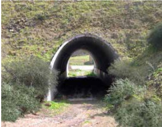
Figure 12.3. Vegetation at the entrance of a multi-use crossing that provides shelter for animals. Photo: Minuartia.
