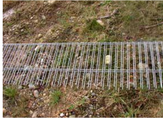
Figure 13.6. Detail of welded wire mesh reinforcement. Photo: C. Rosell.
