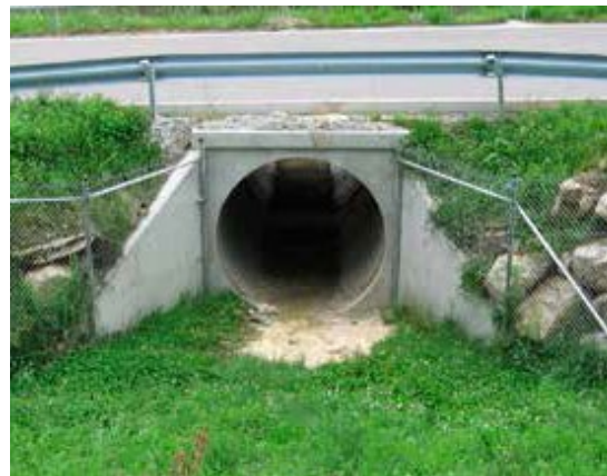
Figure 12.6. Correctly installed perimeter fencing. Photo: M. Fernández-Bou.
