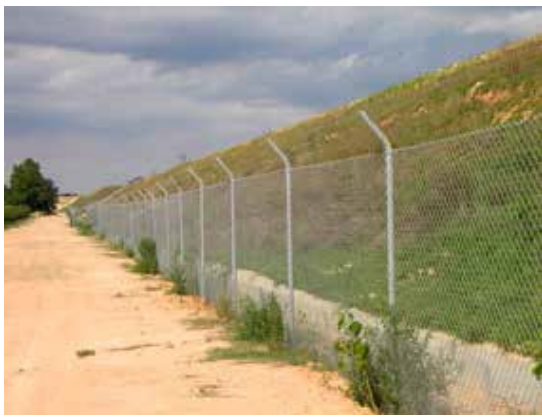
Figure 13.2. Fence set at the base of an embankment. Photo: F. Navàs.
