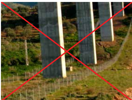
Figure 5.9. Long section of perimeter fencing under a viaduct which prevents animal passage. Photo: Minuartia.
