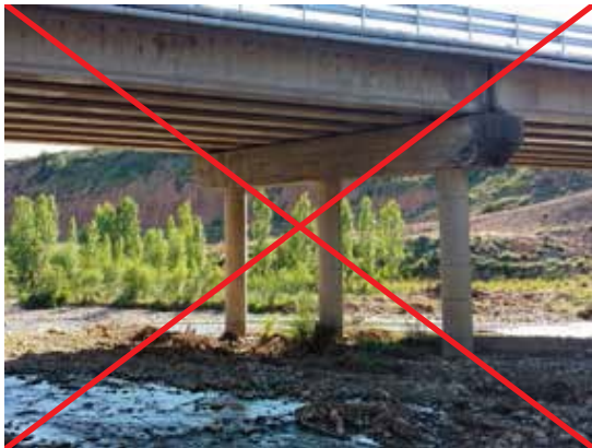
Figure 5.7. Incorrect location of viaduct piles in the watercourse. Photo: F. Navàs.
