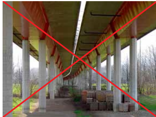
Figure 5.8. Inappropriate use of land beneath a viaduct. Photo: C. Rosell.
