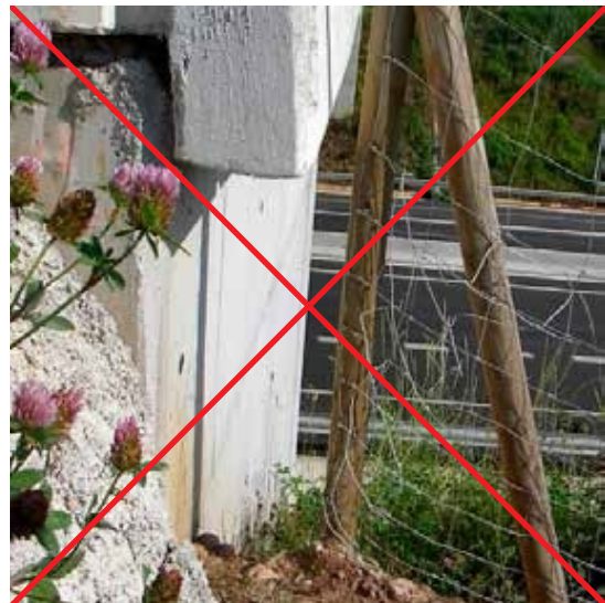
Figure 13.13. Bad adjustment between a fence and an overpass abutment. Photo: F. Navàs.
