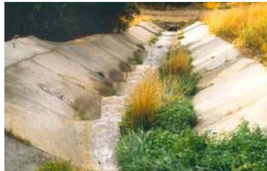
Figure 9.8. Protective culvert outlet on an embankment with sloping side walls adapted to facilitate movement by wildlife. Photo: C. Rosell.
