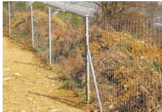
Photo: Roads Department, Government of Madrid.
