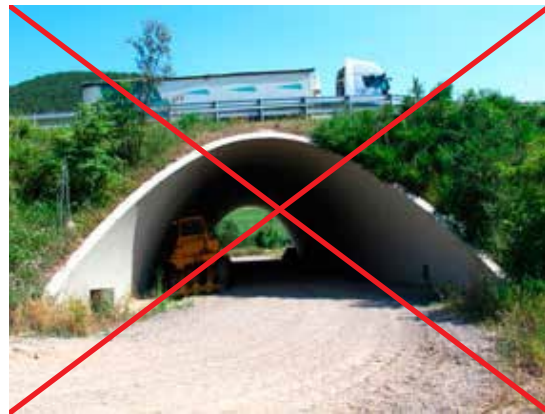
Figure 7.8. Inappropriate use of an underpass to park machinery. Photo: M. Fernández Bou.
