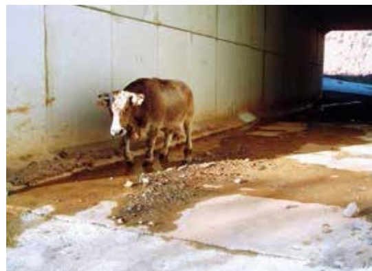
Figure 7.5. Cattle underpasses can also be adapted to facilitate their use by wildlife. Photo: E. Perapoch.
