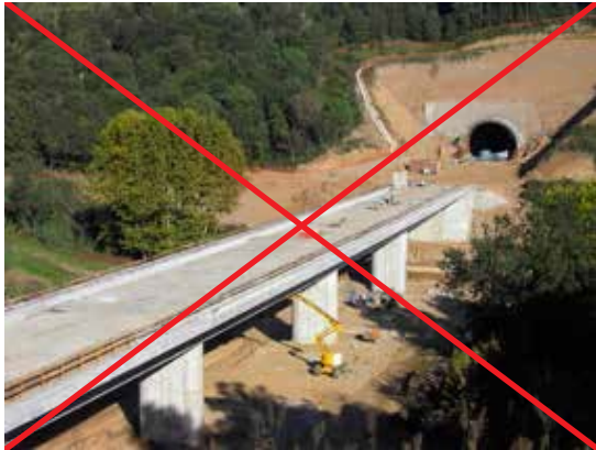
Figure 5.5. Destruction of watercourse habitats during construction. Photo: C. Rosell.
