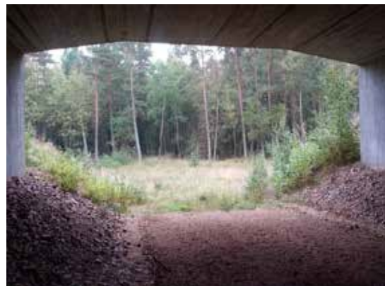
Figure 6.3. Natural soil underpass base. The lack of light and moisture do not allow vegetation growth inside the structure. Photo: C. Rosell.
