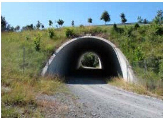
Figure 7.4. Unpaved track and fence tied in with the underpass wing walls encourages wildlife usage. Photo: M. Fernández Bou.
