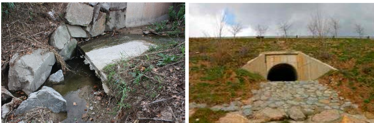
Figure 2. Eroded exit of a drainage. It is usual that culvert accesses degrade due to water erosion of natural substrate creating steps or significant height difference between the concrete base of the transversal structure with the adjacent land. Continuity could be restored by construction stone bed ramps at the exists of culverts. Photos: MINUARTIA.
