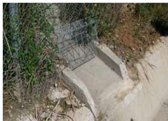
Figure 13.9. Two alternative systems to prevent animal passage at the interface between fences and roadside drains. Photos: Minuartia.
