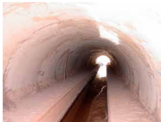
Figure 9.4. Interior of a culvert with dry lateral ledges. Photo: F. Navàs.
