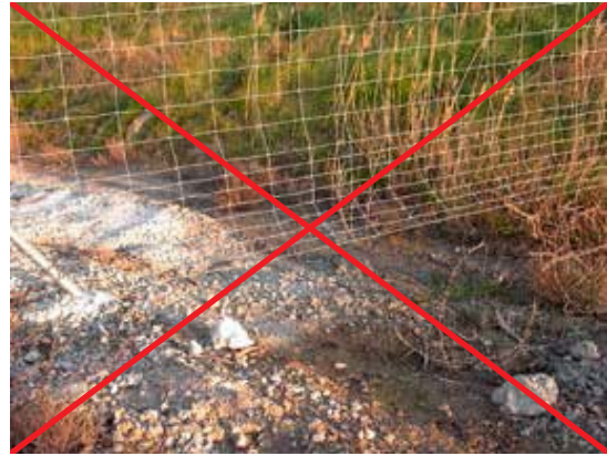
Figure 13.11. Unburied mesh that has been raised by animals. Photo: F. Navàs.
