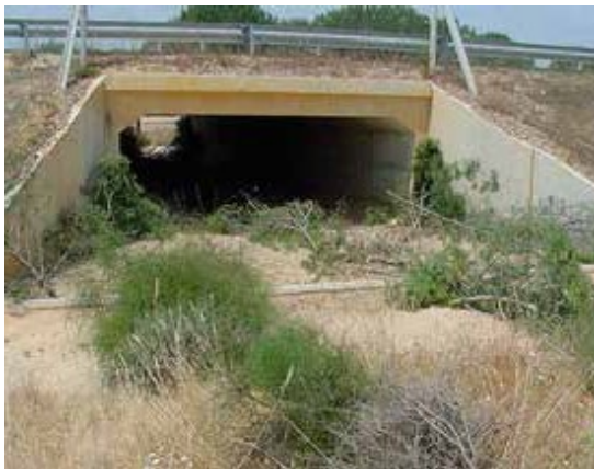
Figure 12.5. Rows of branches and revegetation helps to guide wildlife into the structure. Photo: P. Robles.
