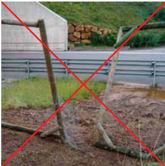
Figure 13.12. Lack of maintenance facilitates wildlife entrance to a road. Photo: F. Navàs.
