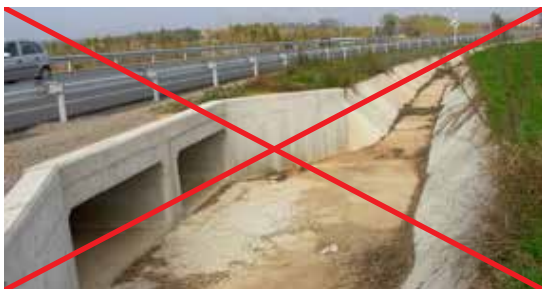
Figure 9.9. Canal fences prevent animals from returning to the surroundings. Photo: F. Navàs.
