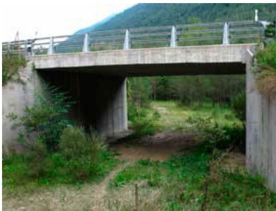
Figure 6.4. Revegetation facilitates the integration of the underpass with its surroundings. Photo: Territory and Sustainability Department, Government of Catalonia.
