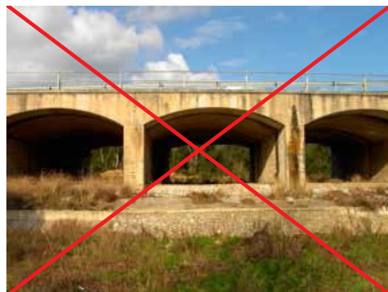
Figure 5.10. Bridge with a concreted zone underneath that prevents the continuity of the riparian vegetation. Photo: Minuartia.
