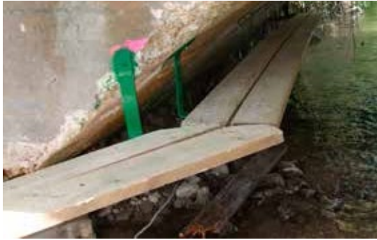
Figure 9.5. Platform that facilitates animal movement through a culvert. Photo: Development and Environment Department, Government of Castilla y León.
