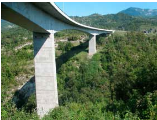
Figure 5.3. Viaduct that allows a complete continuity of forest and riparian habitats. Photo: C. Rosell.
