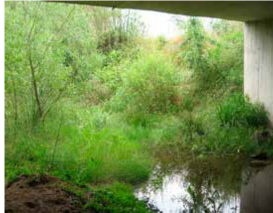
Figure 12.4. Continuous natural vegetation to the entrance of a modified culvert crossing helps to guide animals and increases the use of the structure. Photo: M. Fernández Bou.
