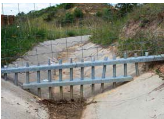
Figure 13.9. Two alternative systems to prevent animal passage at the interface between fences and roadside drains. Photos: Minuartia.
