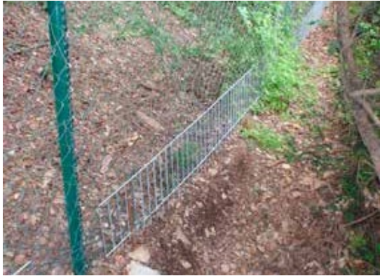
Figure 13.5. Wild boar reinforcement in a particularly troublesome section. Photo: Túnel Barcelona-Cadi.
