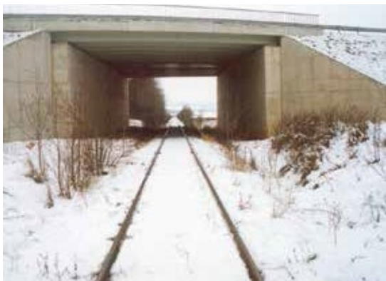
Figure 7.2. Railway underpass used by low-frequency rail traffic and wildlife. Photo: V. Hlavac.
