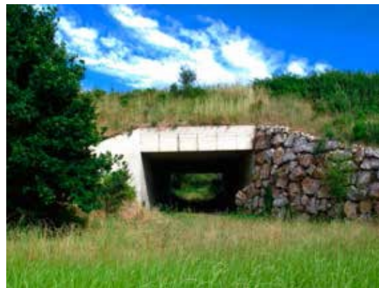
Figure 6.5. Structure with well adapted entrance. Photo: M. Fernández Bou.
