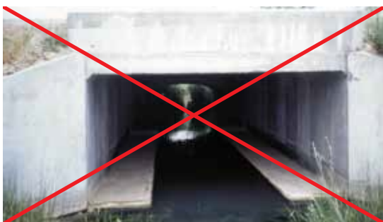
Figure 9.10. Lack of ramps connecting the dry ledges with the adjacent areas. Photo: F. Navàs.
