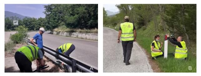
Figure 5.2. Installation of the Virtual Barrier emitters of sound and light on a road safety barrier (A) and in road posts (B). Photo by LIFE SAFE-CROSSING.
