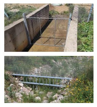
Figure 8.16. Special adjustments must be provided in the intersection of fencing with perimeter drainage ditches. Photos by: Egnatia Odos SA and Minuartia.
