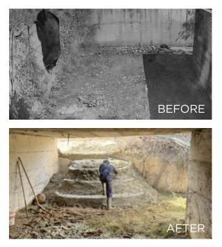
Figure 8.11. 'Before and After' the construction of a ramp to allow bears to overcome a wall at he entrance of an underpass. Photos by: Egnatia Odos SA.
