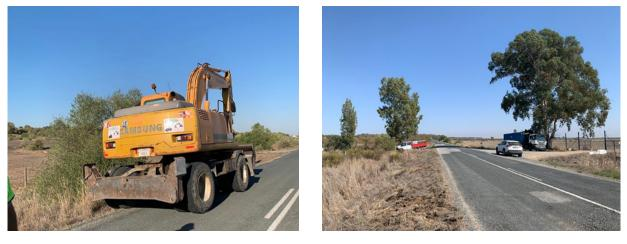
Figure 7.1. Strip of verge cleared to allow visibility of wildlife beside the road. This type of management could also benefit species of vegetation and invertebrates and reduce the risk of forest fire propagation Photo by: Junta de Andalucía.
