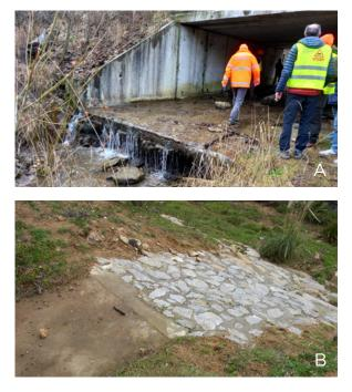
Figure 8.10. A variety of obstacles for wildlife can be found at the entrance of structures such as big steps (left) which could be modified providing stone bed ramps (right). Photos by: LIFE SAFE-CROSSING.
