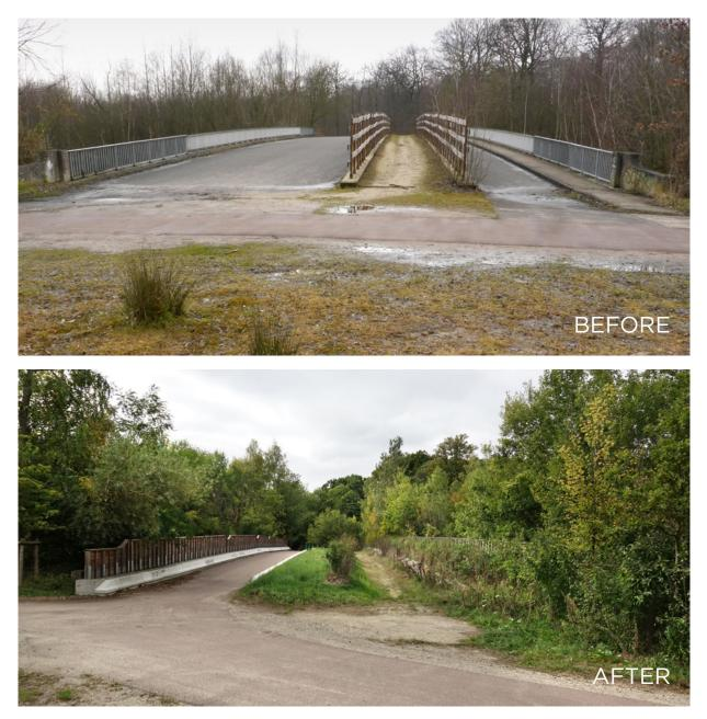
Figure 8.3. Example of upgrading an overpass to a multiuse wildlife overpass. Works consist on providing vegetated strips and installing screens to reduce disturbance from traffic under the passage. All crossing structures with suitable features located in a conflictive road section can be upgraded at moderate costs. Photos by: Jean Luc Barrallier and Vicent Vignon.
