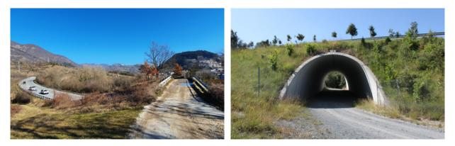
Figure 8.1. Many existing structures (over and under linear transport infrastructure) may be adapted to increase their use by fauna becoming multiuse wildlife passages. These structures can combine wildlife crossing function with other uses such as drainages, cattle trails or forestry roads. Photos by: Minuartia; LIFE SAFE-CROSSING.
