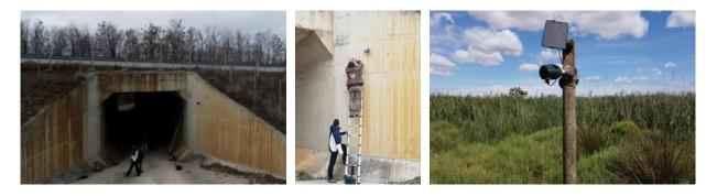
Figure 8.17. Installation of the devices in underpasses to be monitored. The 4G wireless camera including a solar panel were installed. Photos by: Callisto; Cosmote; Minuartia.
