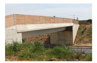
Figure 8.9. Opaque screens allow to reduce disturbance from traffic at wildlife passages. Photo by: Minuartia.
