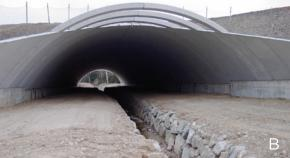
Figure 8.8. Ledges at both sides of drainages can be useful for providing dry passages to small and medium size fauna. An alternative solution to upgrade underpasses for large mammal is to dig a ditch along the central part of the drainage (an example under construction is shown at right). Photos by: (A) Courtesy of the IENE Biodiversity and Infrastructure online handbook; (B) Minuartia.
