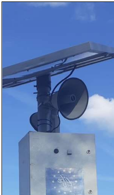
Figure 10. Loudspeakers above the electrical box of the central unit (Terni Province).
