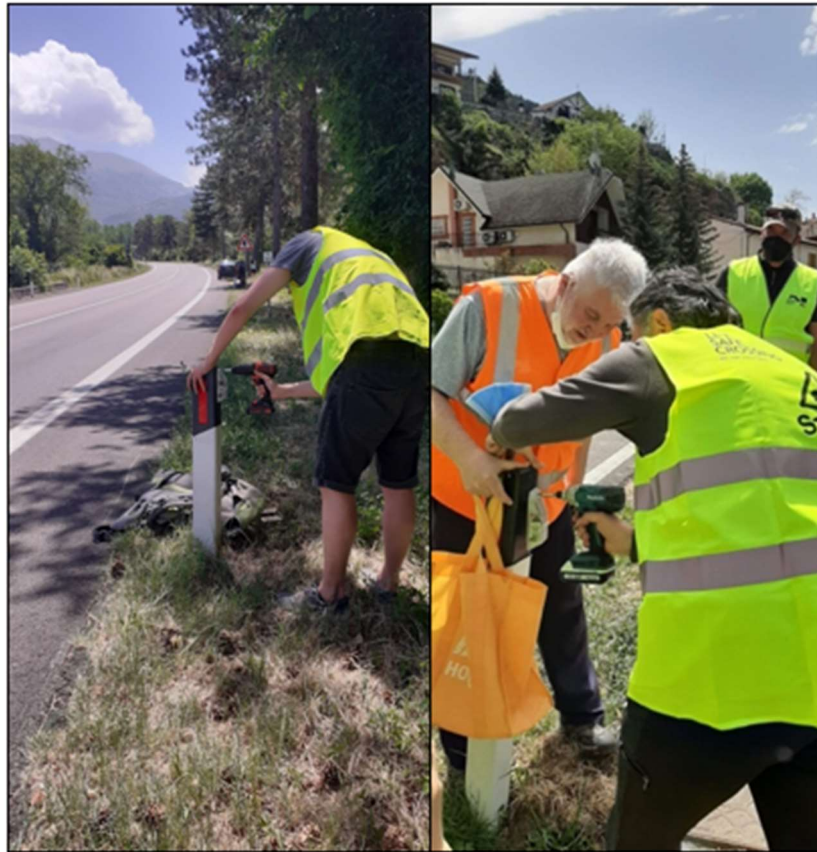
Figure 16. Installation of the VF unit on the road post in PNM on the left and in PNALM on the right.
