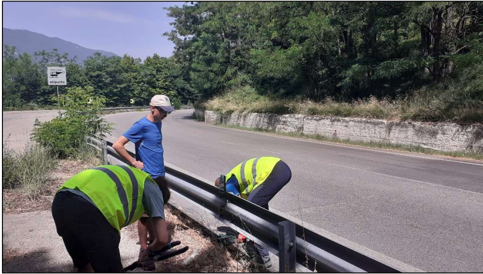
Figure 18 Installation of the VF device on guardrail in PNM.
