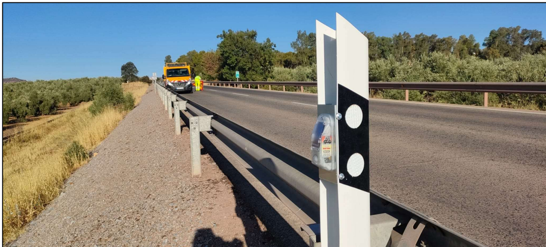
Figure 14. Unit of the virtual fence installed on a road post in Spain.
