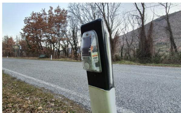
Figure 5.1. Virtual Barrier emitter units installed on road post in Spain and Italy. Photo by LIFE SAFE-CROSSING.
