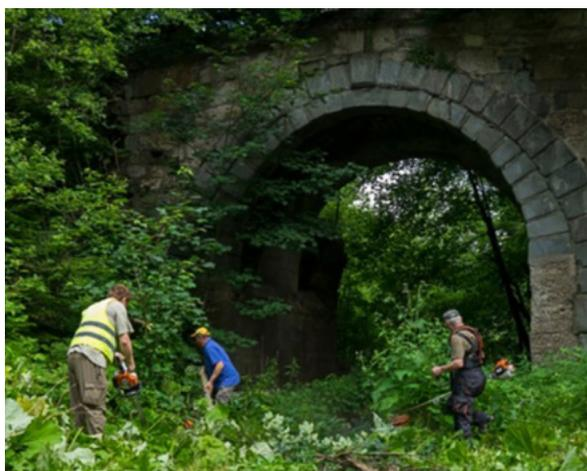
Figure 8.13. Vegetation allows to avoid erosion in embankments and to guide animals through the passage entrance. Local species are used for re-vegetation. Photos by: LIFE SAFE-CROSSING.
