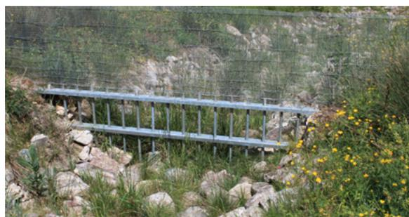
Figure 8.16. Special adjustments must be provided in the intersection of fencing with perimeter drainage ditches. Photos by: Egnatia Odos SA and Minuartia.
