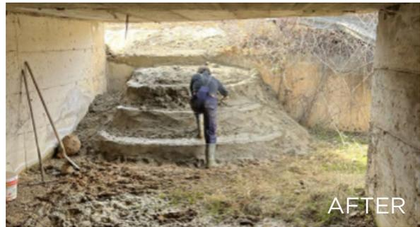
Figure 8.11. 'Before and After' the construction of a ramp to allow bears to overcome a wall at the entrance of an underpass. Photos by: Egnatia Odos SA.
