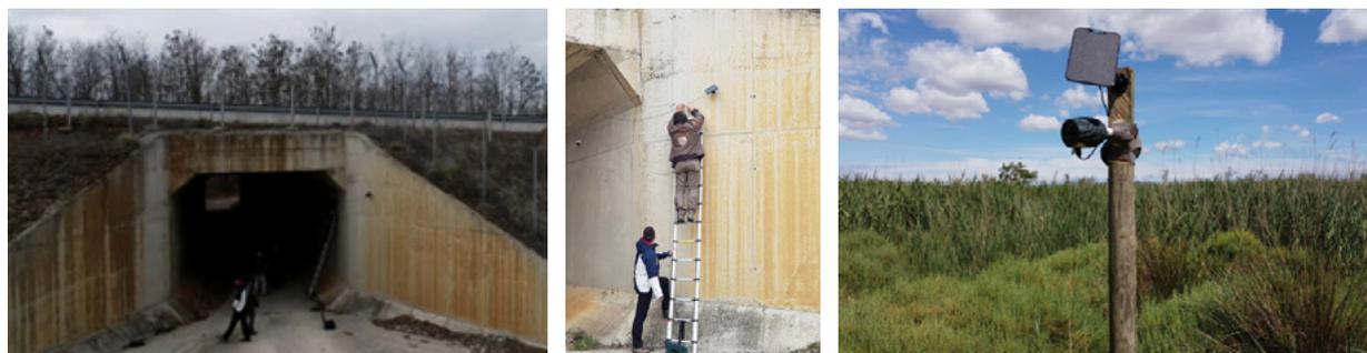
Figure 8.17. Installation of the devices in underpasses to be monitored. The 4G wireless camera including a solar panel were installed. Photos by: Callisto; Cosmote; Minuartia.
