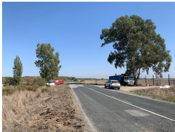
Figure 7.1. Strip of verge cleared to allow visibility of wildlife beside the road. This type of management could also benefit species of vegetation and invertebrates and reduce the risk of forest fire propagation
