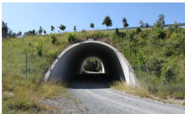
Figure 8.1. Many existing structures (over and under linear transport infrastructure) may be adapted to increase their use by fauna becoming multiuse wildlife passages. These structures can combine wildlife crossing function with other uses such as drainages, cattle trails or forestry roads. Photos by: Minuartia; LIFE SAFE-CROSSING.
