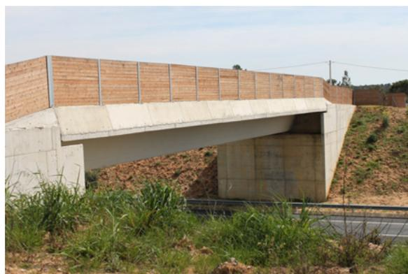
Figure 8.9. Opaque screens allow to reduce disturbance from traffic at wildlife passages. Photo by: Minuartia.
