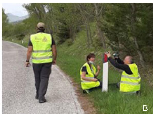
Figure 5.2. Installation of the Virtual Barrier emitters of sound and light on a road safety barrier (A) and in road posts (B). Photo by LIFE SAFE-CROSSING.
