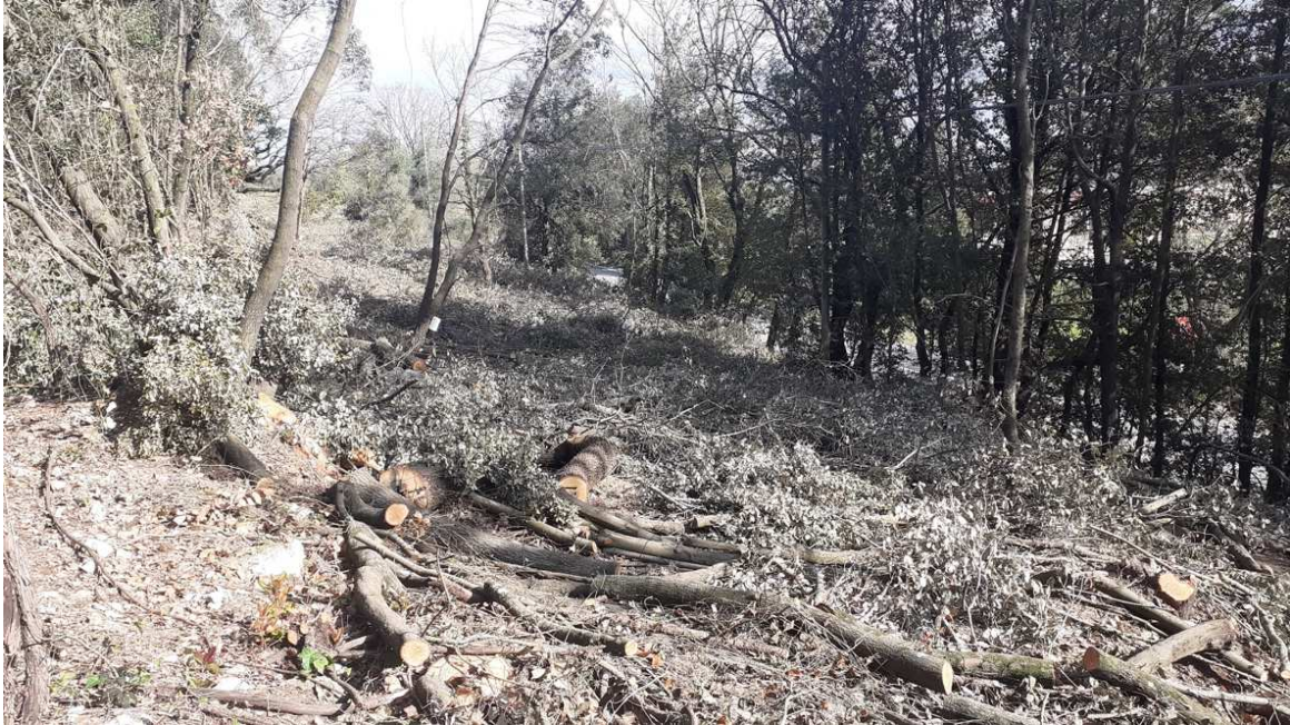
Figure 11. Forest cutting operation in the area of the AVC-PS Amelia 2 in Terni Province (the white device is a PIR sensor).
