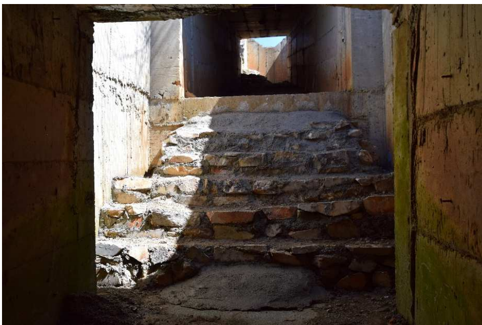
Figure 44. Construction of stairs in the culvert K73 in the A29 Highway (Photo by L. Georgiadis).
