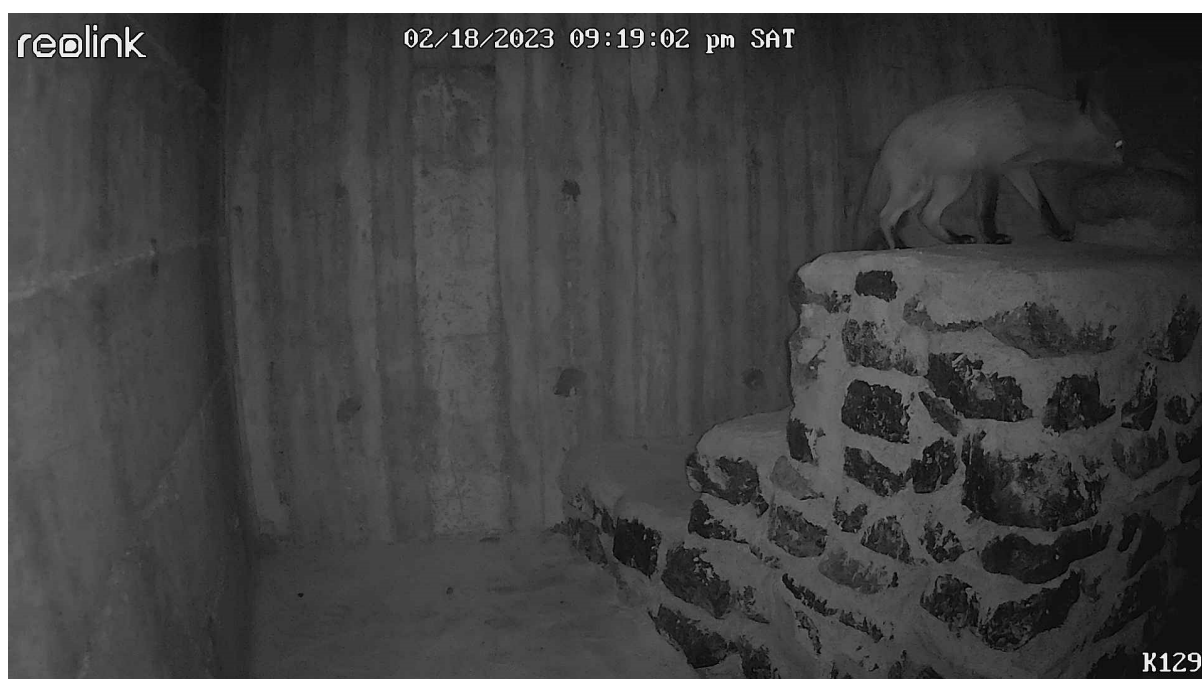
Figure 45. A fox using the new constructed stairs inside of the culvert K129 in the A29 Highway recorded by the camera of COSMOTE.
