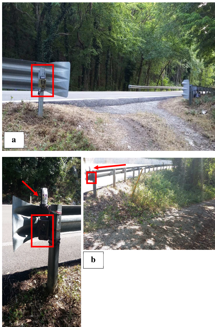
Figure 3. Solution found to install camera traps preventing the vehicles from triggering the cameras themselves: cameras are installed behind the guard rail that works as a shield between vehicles and the camera sensors. Red squares highlight the camera traps while red arrows highlight VF devices in: a) One camera trap along the SS5 before the installation of the VF; b) camera traps along the SS487 after the installation of the virtual fence. The lockers and the special anti-theft covers are clearly visible in the picture a.
